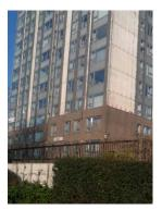
Chalcots tower with cladding removed showing the original concrete panel finish
