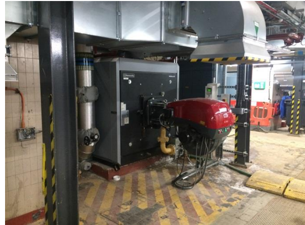
Replacement boiler plant installed in 2017
