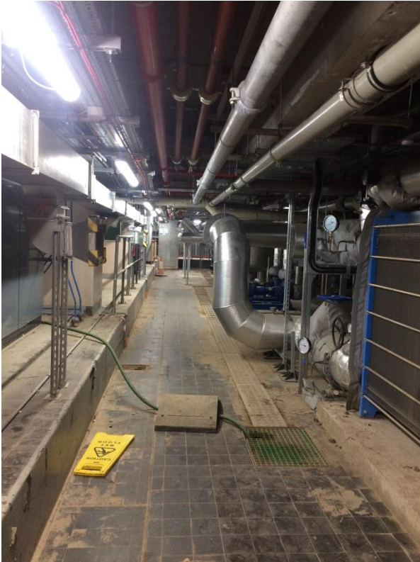
Plant rooms contain asbestos both in the containment lining and fabric of the structure
